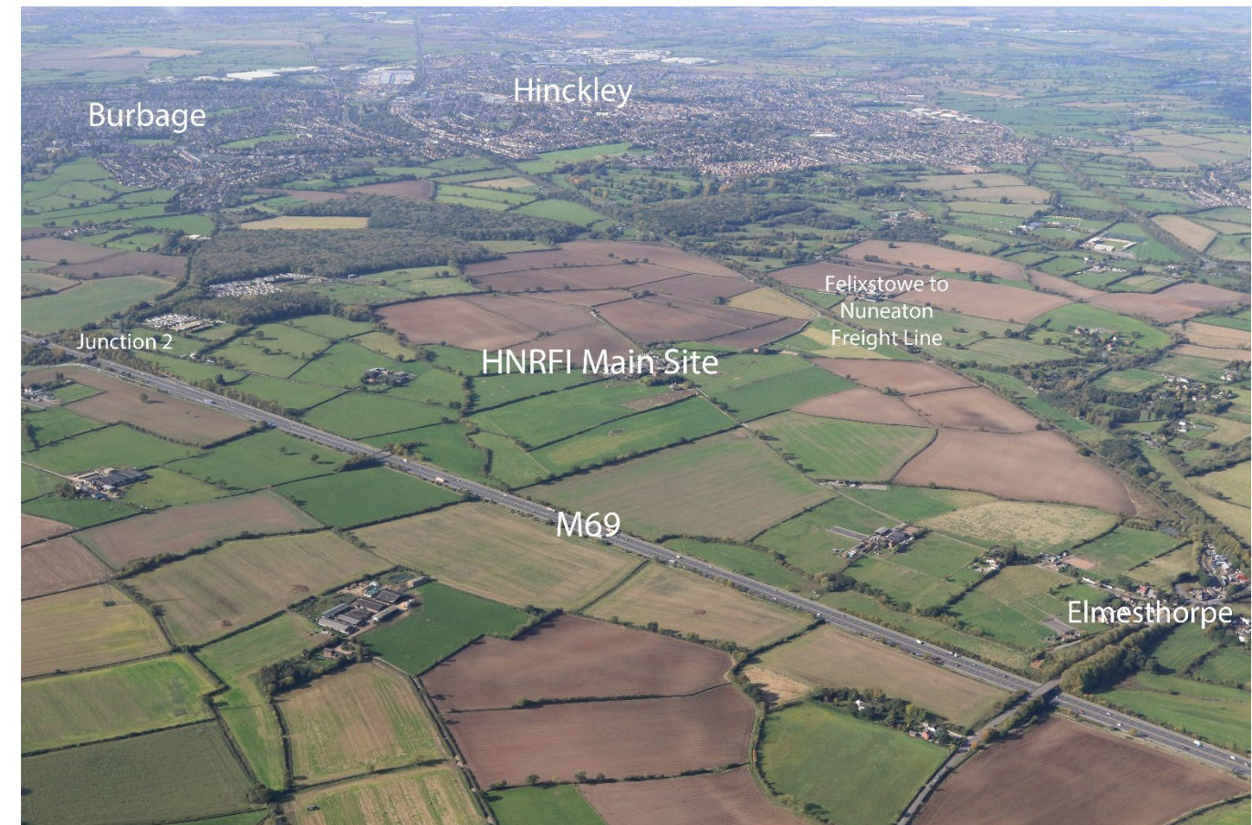
Fig.5 Aerial image of Main HNRFI site with M69 in foreground looking towards Hinckley and Burbage
